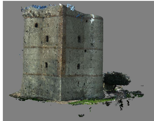
Fig. 4 Dense Point Cloud
