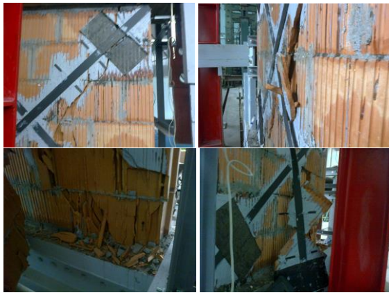
Fig. 5 Failure mode for URM1-C (URM1-strengthened)
